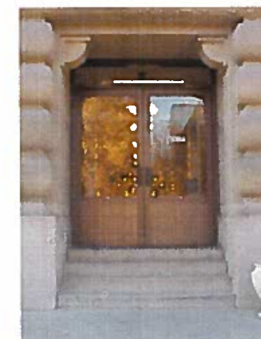
The north entry doors have been replaced with bronze anodized aluminum.
