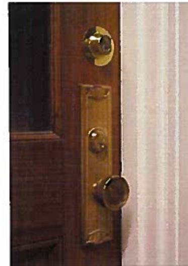
Some of the hardware and screws are missing at various locations. Some hardware is mismatched.
