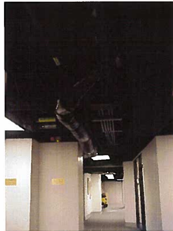
The ceilings in the basement near the rotunda have excessive amounts of conduit, piping and ductwork exposed to the area. Consideration should be given to removing or relocating these elements.
