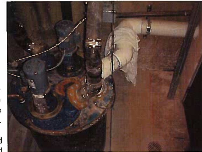
Storm drainage discharge into sewage ejector
