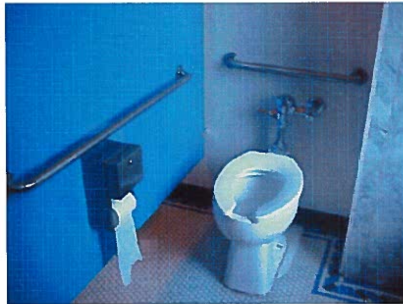
Finishes in the public toilet rooms are varied. The first and second floor men's rooms have retained the original floor tile. The original marble toilet partitions have been replaced with metal partitions (left, first floor men's toilet room).
