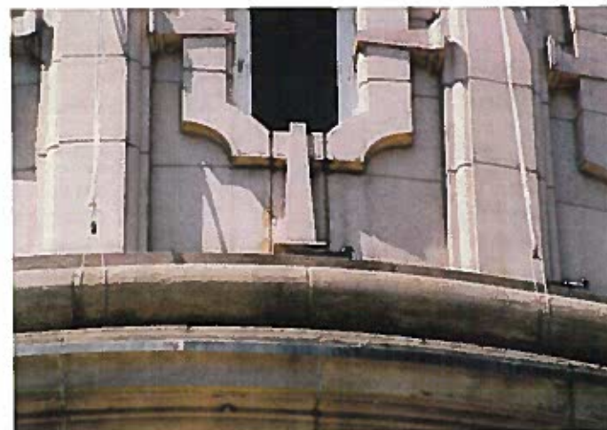
Approximately 10 small spalls were observed in the surface of the terra cotta dome. Most of these spalls occur at the corners of ornament and are less than 2 inches in diameter.
