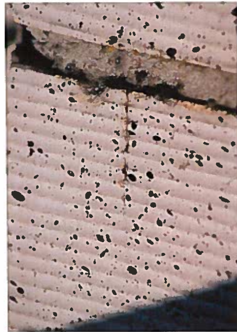
Minor cracks were observed throughout the exterior walls, drum and dome, mainly at the cornice and at corners of window openings. Some cracks have been filled with sealant or mortar. Approximately 10 minor cracks were observed in the terra cotta dome.
