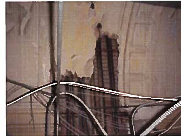
Most plaster elements above lay-in ceilings have been severely damaged by the installation of mechanical, electrical and ceiling systems. Upper portions of wood window casings have also been damaged by the installation of lay-in ceilings.
