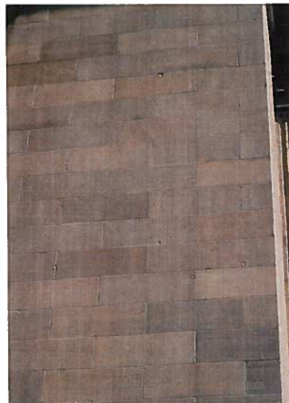
Several regions of shallow spalls were identified on sandstone units. The spalls are typically less than 1 inch deep and are only visible when shadows are cast in the spalls.
