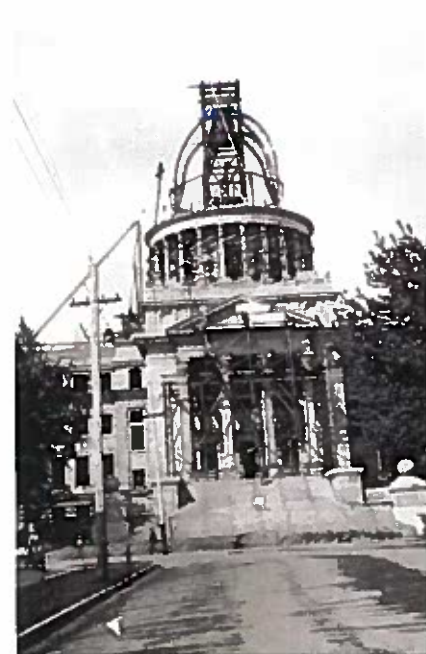
Layer upon layer, the dome rose above Boise in 1912. The sandstone columns of the peristyle encircle the dome's steel drum, and above this the structural members of the dome begin to suggest the soaring height of the completed building.
