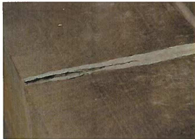
Sealant joints at the water table are typically deteriorated and have exhibited cohesive failure. Sealant joints at the parapet and terra cotta dome were observed to be in good condition.
