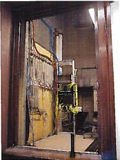
Data and telecommunications systems equipment, cabling, wiring and panels have been installed in former light shafts, elevator shafts or other "found" spaces throughout the building.
