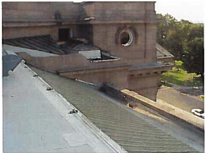
The decorative green glazed clay tile visible from the south is in good condition. Several rows along the lower edge of the tile have been removed and replaced with single-ply roof flashing to aid drainage.
