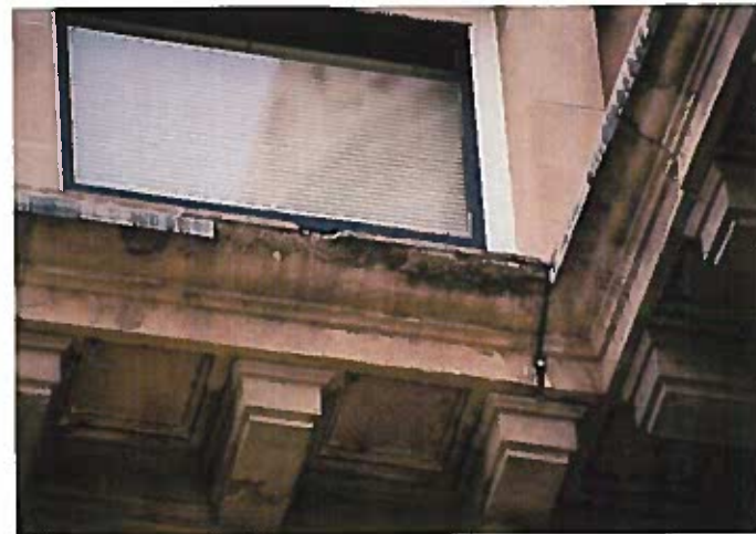
Only a few deep spalls (greater than 1 inch deep) were observed in sandstone units. Locations of deep spalls correspond to areas of maximum weather exposure such as the parapet and cornice and areas with missing flashing.
