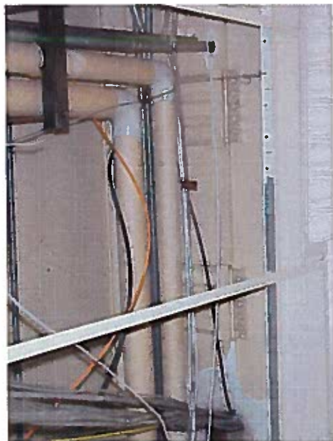
Initial installation and relocation of data and telecommunications systems cabling has been randomly placed and, when abandoned, left in place.
