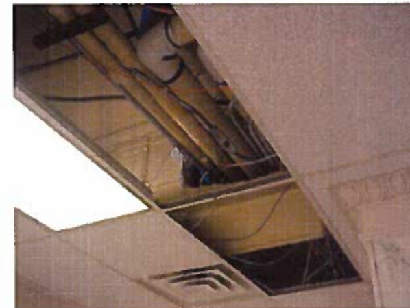
Consideration should be given to removing lay-in ceilings in areas with original decorative ceiling elements.
