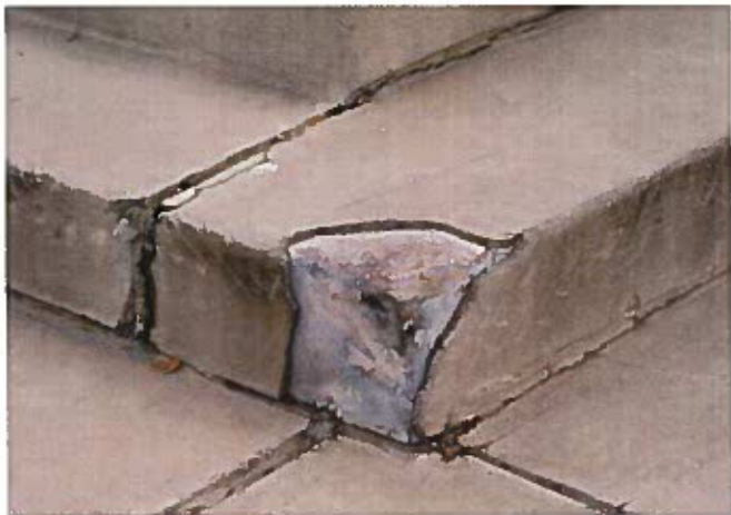
The concrete topping slab on the east and west stairs is deteriorated in several locations, presenting a tripping hazard as well as allowing the penetration of moisture into the structure below.
