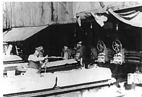
Rock was cut into coarse blocks at Table Rock Quarry and transported to the Capitol construction site, where it was finished and readied for placement.
