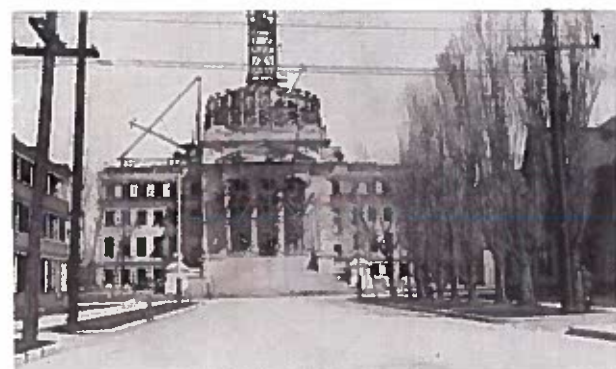
The steel skeleton of the dome's drum, or supporting cylindrical base, takes shape as the south entrance portico is completed.
