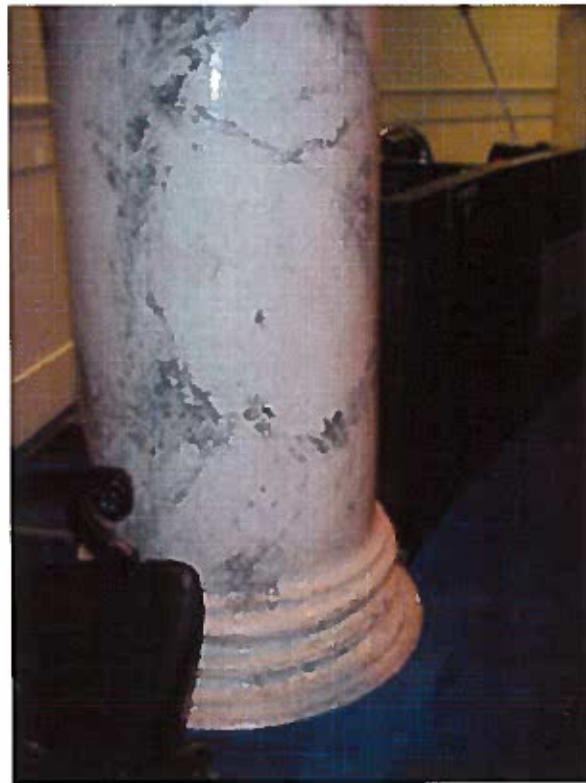
Columns currently show signs of aging, displaying hairline cracks in various degrees of severity. The columns in the House (above) and Senate chambers appear to have more cracks than the columns in the rotunda due to higher use and abuse with furnishings.
