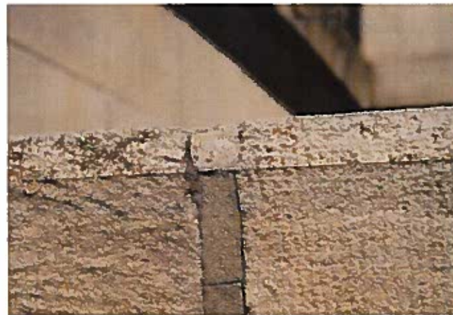
Most of the mortar joints at the walls and drum were observed to be in good condition. Joints at the cornice and parapet level of the walls and the entry pavilions are most deteriorated. Some mortar joints show evidence of re-pointing.
