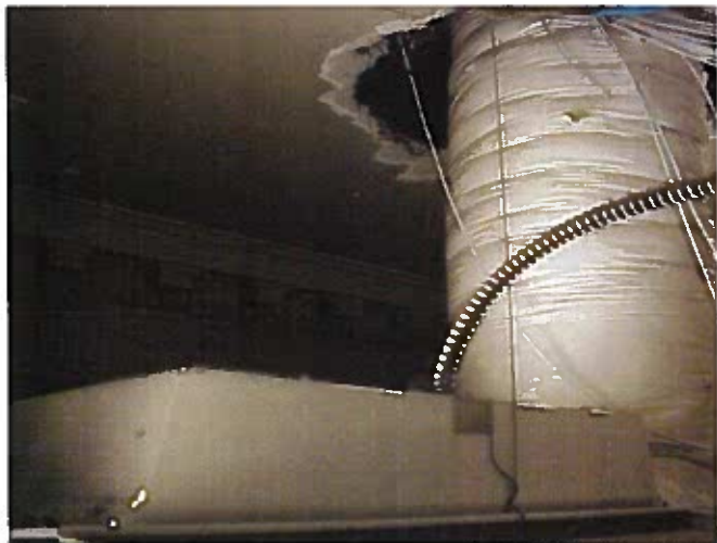
The intent of the building survey is to identify original and non-original materials throughout the Capitol and assess their condition. Hidden behind dropped ceilings, historic moldings and plaster have been damaged to accommodate the installation of modern mechanical systems.
