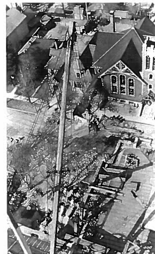
Derricks, purchased by the state, facilitated construction of the Capitol's central portion. They were used to lift the heavy loads of stone and steel in the construction of the dome.
