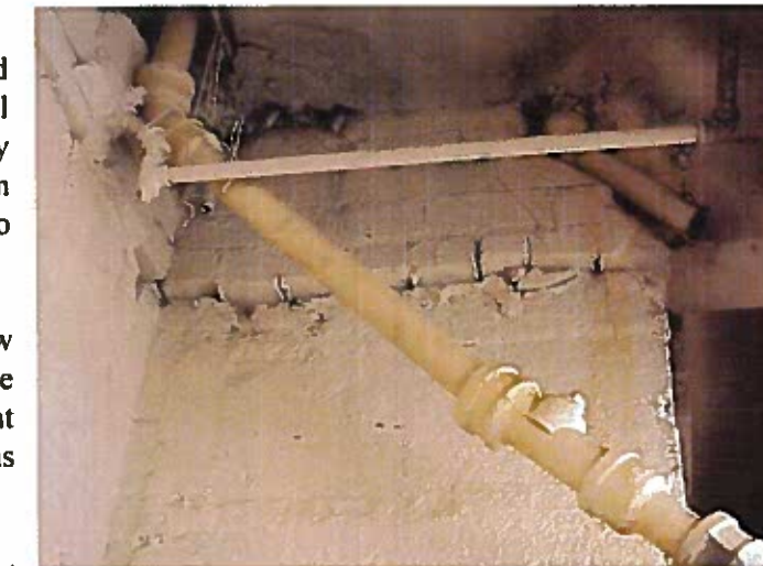
Cast iron sanitary sewer pipe in basement
