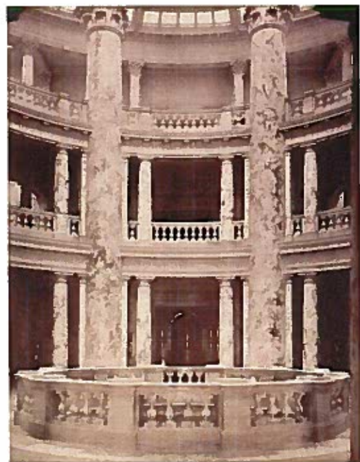
The columns of the rotunda were sheathed with scagliola, a thin decorative coating intended to mimic the appearance of marble. The smaller elements of the balustrades were cut of marble.
