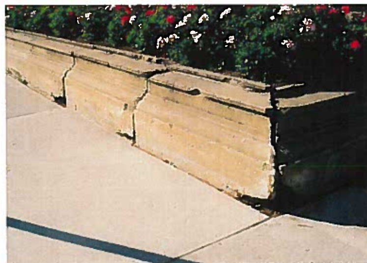
Most of the sandstone planter walls around the perimeter of the building are weathered and spalled. Joints are deteriorated and open. Several units are displaced. These elements may have been subsequently added and may not be original to the 1920 Capitol building completion.
