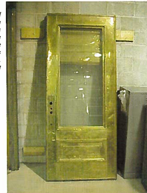
The original exterior doors were built of wood clad in brass. One pair is currently being stored in the Idaho State Historical Society collections warehouse.
