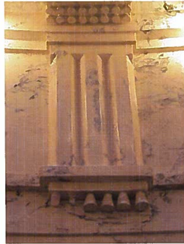
Decorative wall and ceiling triglyphs throughout the building are formed of plaster, wood and marble. Most of the exposed plaster is in good condition; however, numerous pieces and elements are missing or damaged.
