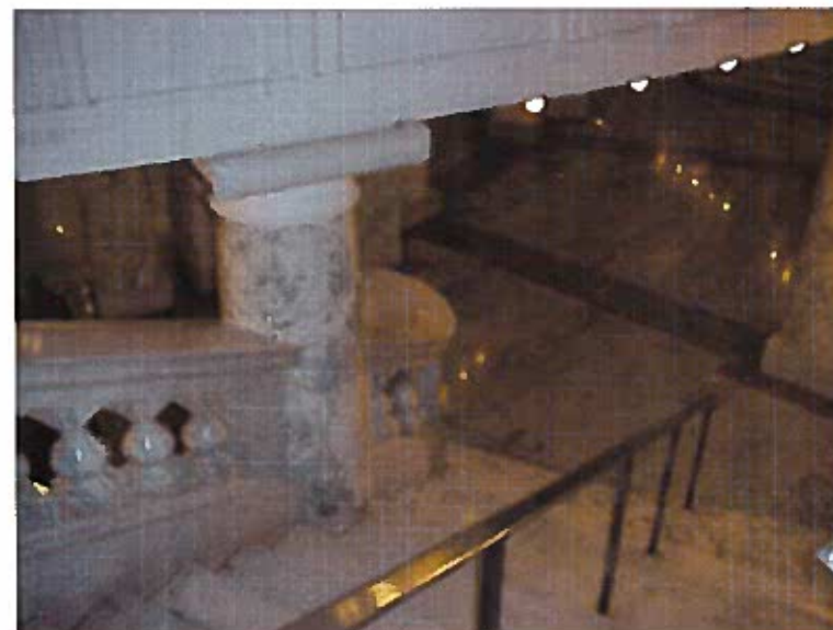
The plaster caps on the top of columns adjacent to the first floor rotunda stairs are retrofit with cushions to protect occupants from injuring themselves on the low projecting corners. Aluminum handrails have been added without proper consideration of original architectural details or materials.
