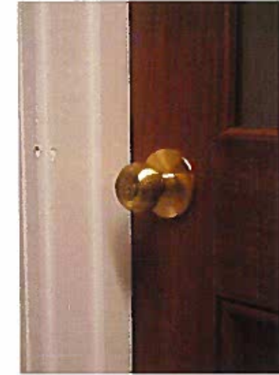
Some of the hardware and screws are missing at various locations. Some hardware is mismatched.
