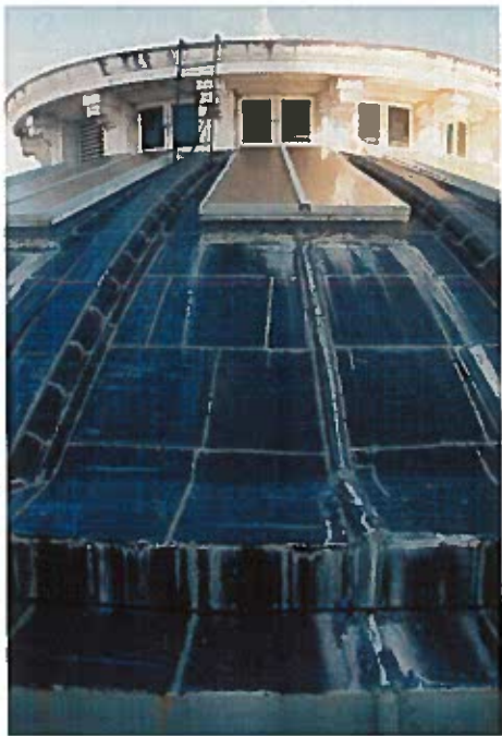
The secondary domes over the House and Senate chambers are clad with copper roofing. The upper portion of the dome is weathered with a light green color. The lower portion of the dome is lead coated, darkly colored with white streaks. The lower roof was originally terra cotta — the terra cotta may still be in place under the copper skin. Skylights in the lower dome have been retrofit with plastic lenses, which appear to be in good repair.
