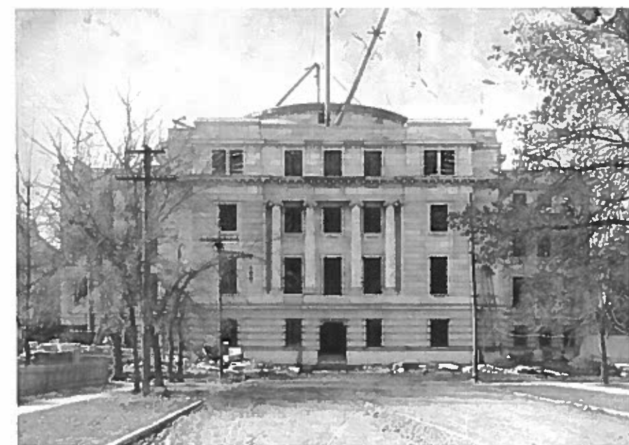
Once the exterior shell of the lower levels of the central portion was nearly complete, work began on the structure of the dome. In this construction photo of the north elevation, the derricks are in place for constructing the dome.
