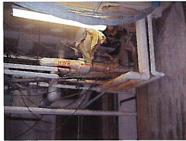
Hot water piping in shaft
