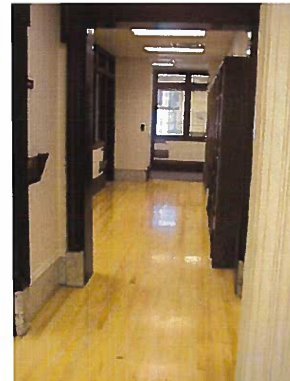
Original maple wood floors are exposed in portions of the first floor Attorney General's office. The wood floors on the east side of the first floor north wing are covered with carpet.
