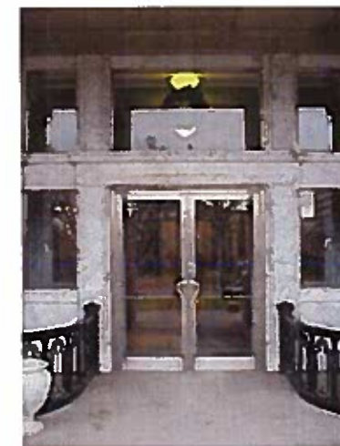
Exterior doors and frames at main entries are stainless steel with the exception of the north entry doors and frames (left, second floor east entry).
