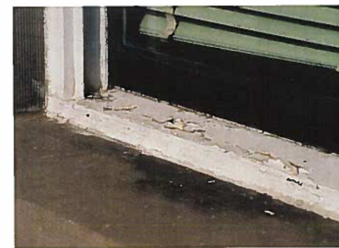
The paint on most windows is peeling. The extent of deterioration varies with exposure and location. Evidence of wood deterioration was not observed.
