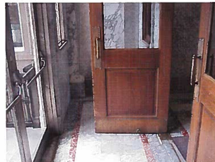
Much of the wood doors and hardware throughout the building are in good condition; however, many of the main entry doors are scratched and worn (left, second floor east entry).
