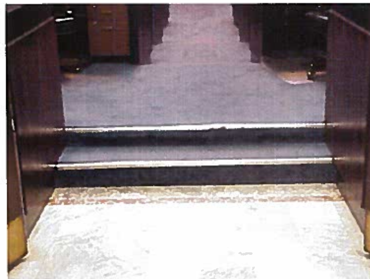
The original cork floors in the House and Senate chambers have been covered by a stepped floor system and carpet.
