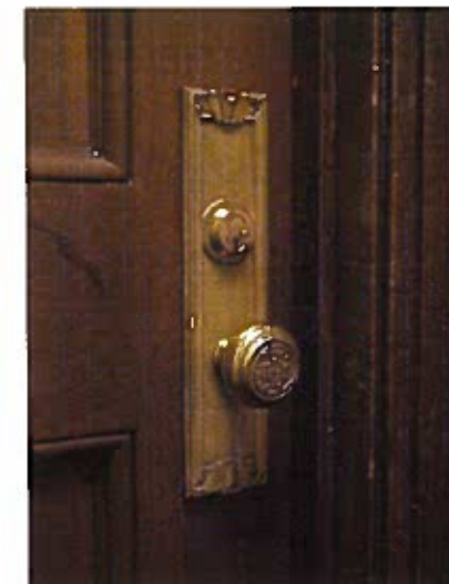
Some of the hardware and screws are missing at various locations. Some hardware is mismatched.
