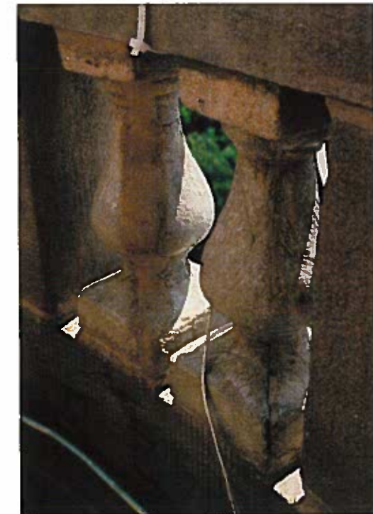
Several of the lantern balusters exhibit characteristics of cast stone, not typical sandstone. Several are eroded and cracked. The casting joint in several is cracked.
